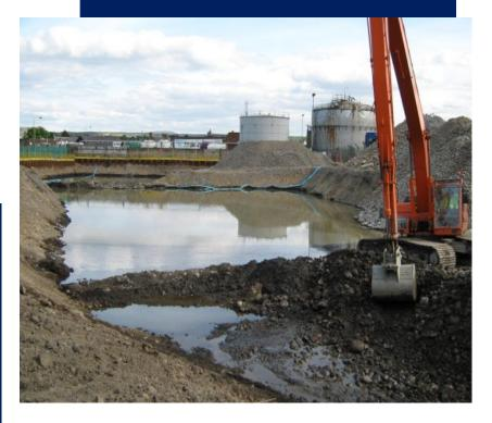
WDE worked alongside the various parties to manage the mass excavation and treatment of diesel impacted hydrocarbon material along with dual phase groundwater treatment. A total of 10,000m³ of impacted material was excavated, screened and treated using thermal desorption remedial techniques. Grossly impacted groundwater was contained using connecting piles and pumped to a groundwater treatment facility onsite. Approximately 3,370 litres of weathered diesel was recovered from groundwater.
